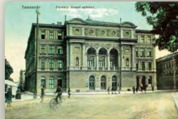
The "Franz Josef" Theater in Timișoara, designed, like that of Chernivtsi, by architects Fellner and Helmer, was inaugurated in 1875.
